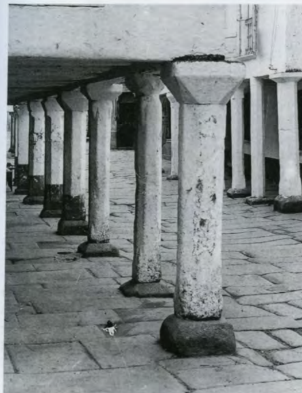
Boundary of a building made by columns and arcades. Notice how each column has its own internal boundaries at the capital and base; and how these two have their own boundaries in the line of detail which bounds them in turn.
