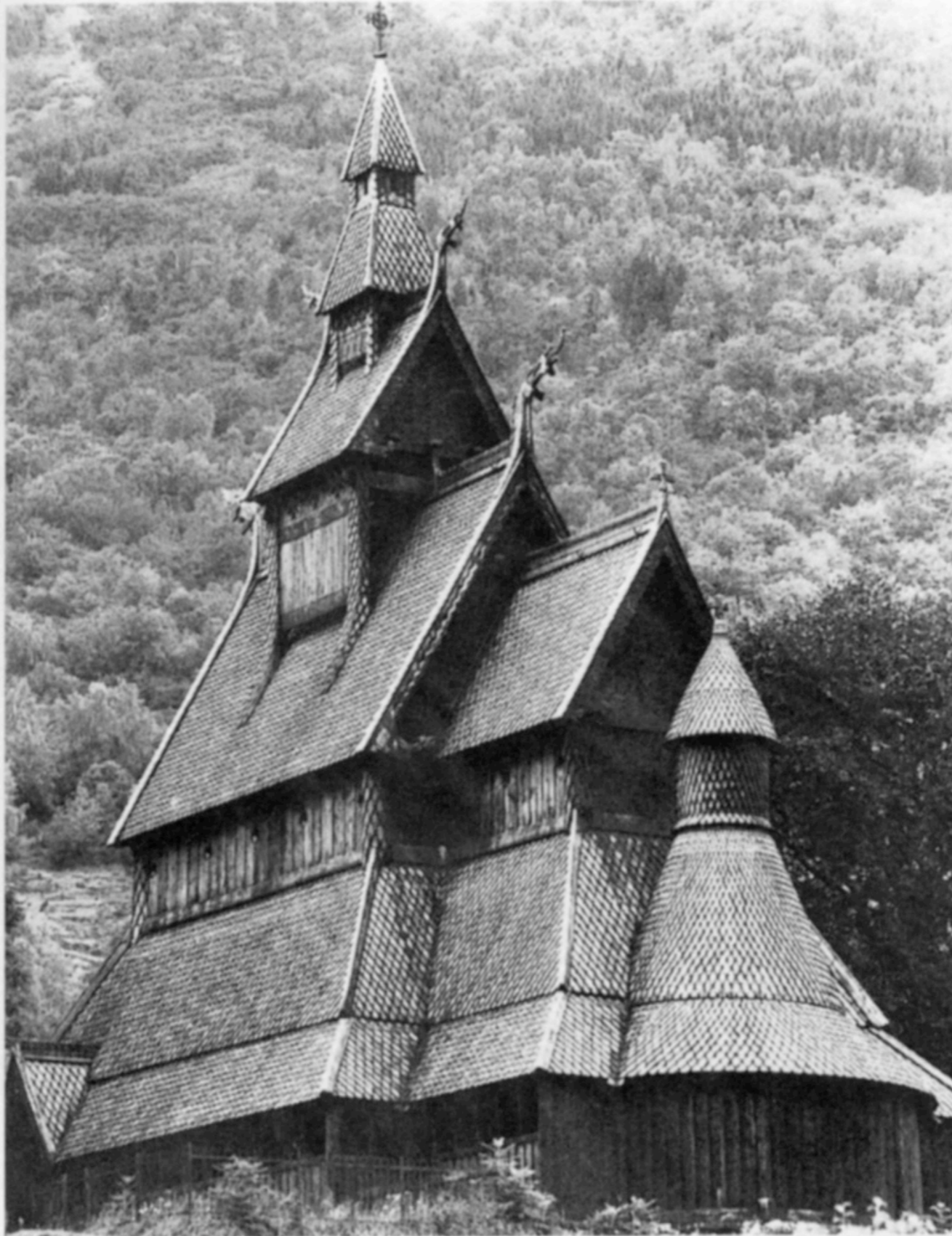
Roofs of a Norwegian stave church
